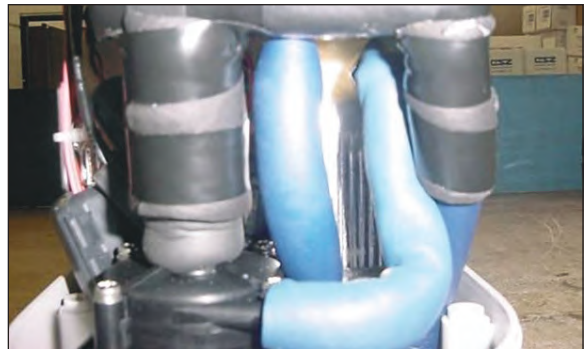
Figure 88 - Step 12 Apply electrical tape around insulation
