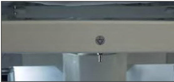
Fig. Potential equalisation connector – male
